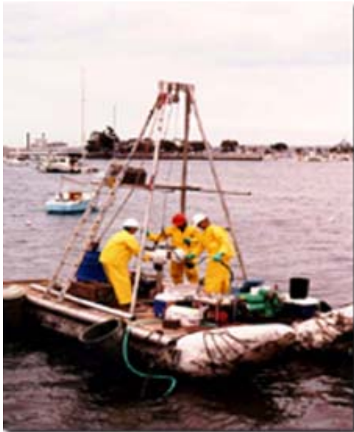
Vibrocoring on Pontoon Barge in San Diego Bay.
